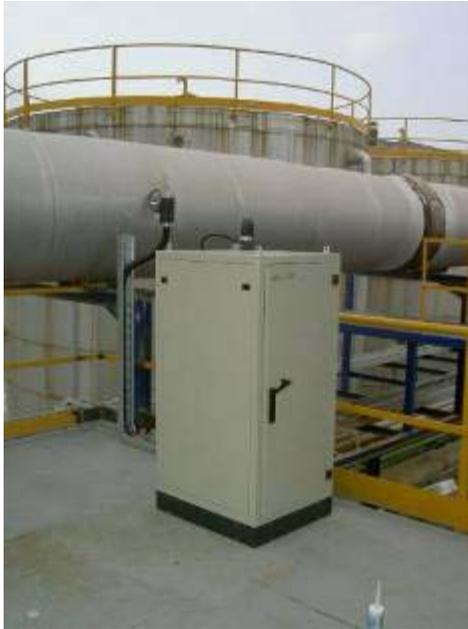
OEM Flue gas analyzer
